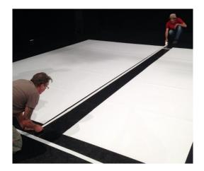
3) Finally place the whole white floor onto the rectangle. Tape it nicely from above with white pvc marley.
